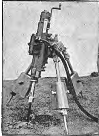
FIG. 172.—Rock-drill.
